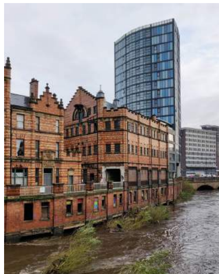
Royal Exchange Buildings, The Wicker
