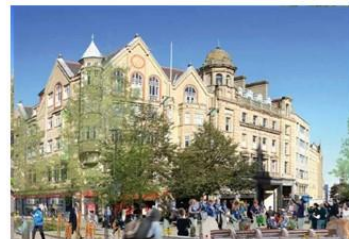
New ground floor doors
